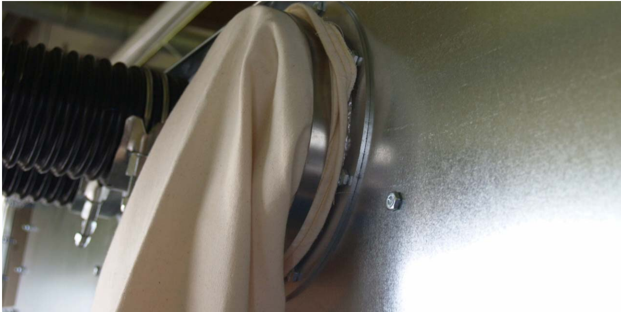
(Photo 7: Installed Filter bag)
