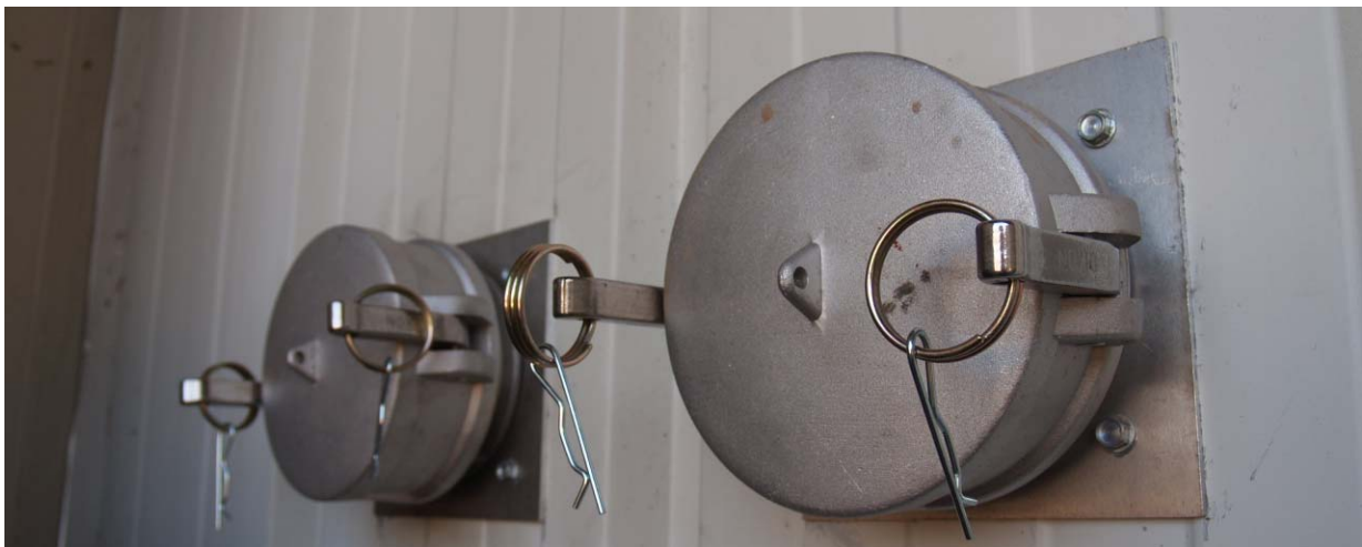
(Photo 3: Installed couplings)
