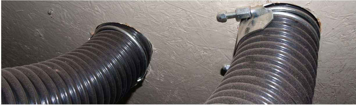
(Photo 4: Spiral clamps used to hold hoses in place)
